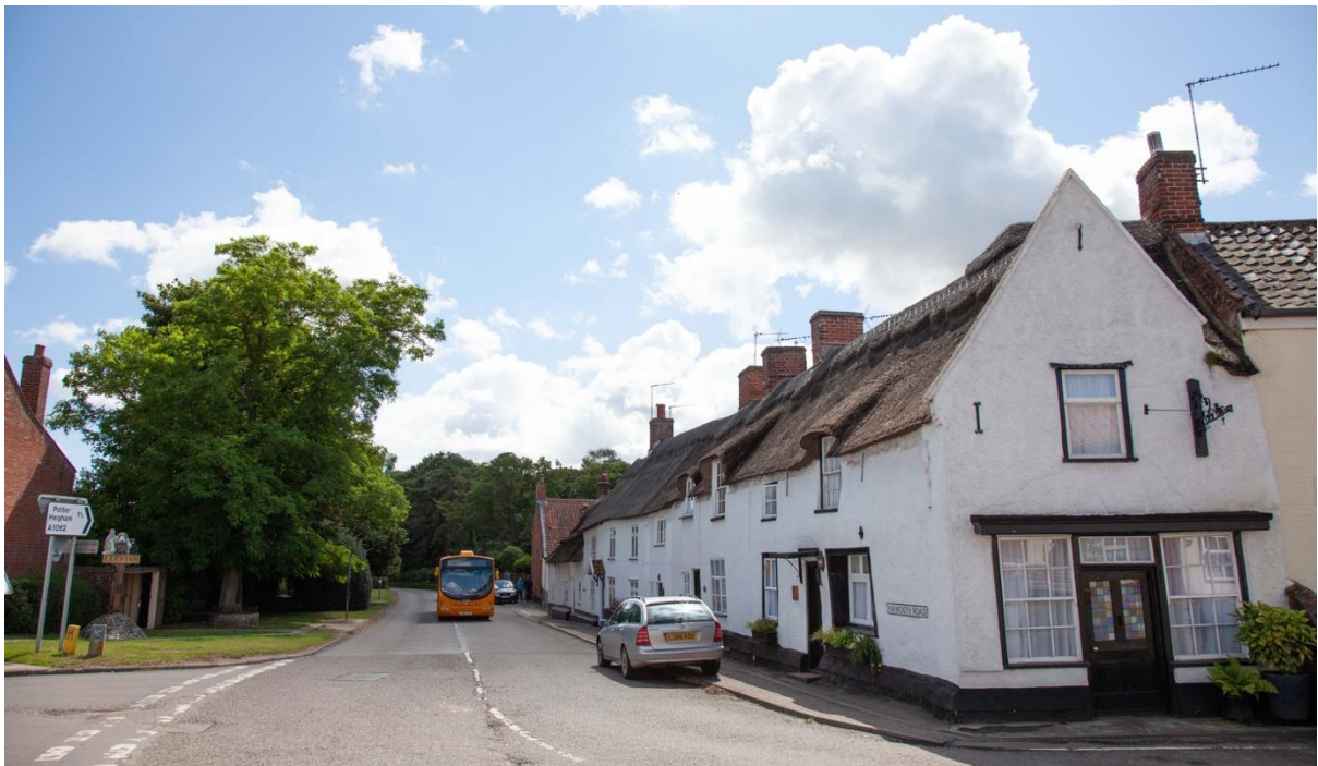
Numbers 1 – 5 on Yarmouth Road are listed
